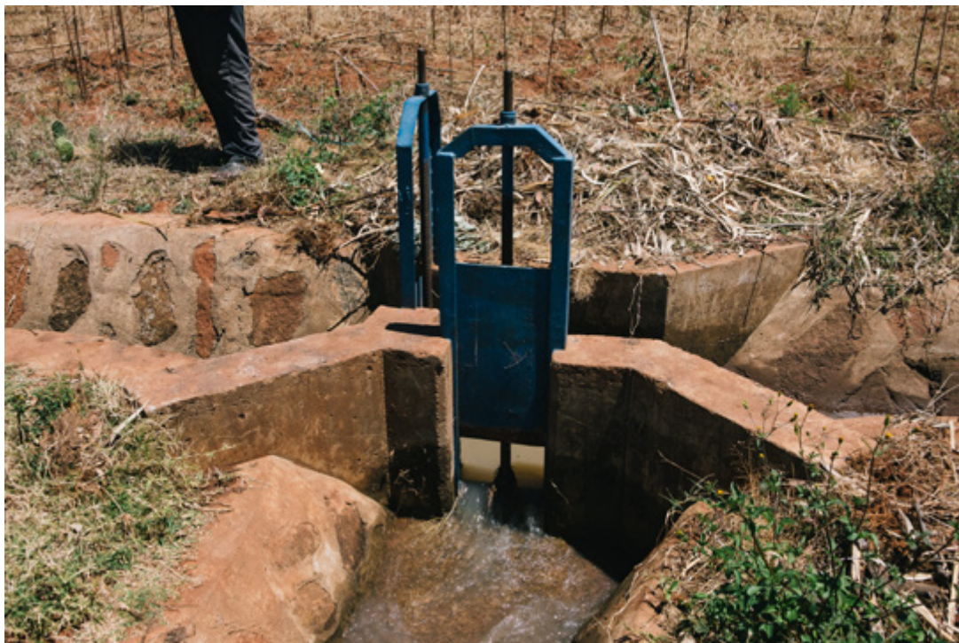
This irrigation system designed by Uniterra volunteers allows the distribution of water to different plots of land.
