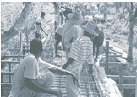
MEN AT WORK BUILDING A RETAINING RESERVOIR. PHOTO BY CECI-HAITI
